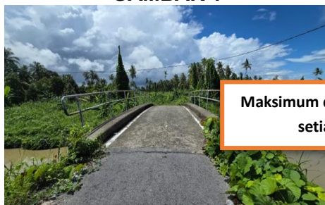
Asajaya IV Drainage Scheme, Samarahan - Concrete Bridge (Bridge 17) (29.11.2024) (Sumber: Unit Audit Dalam)
